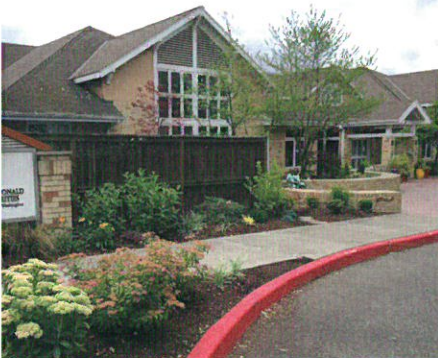
Columbia Construction Services Inc. worked with GAF and Allied Building Products Corp. to help a $1.4 million remodeling project at Ronald McDonald House Charities come to fruition.
